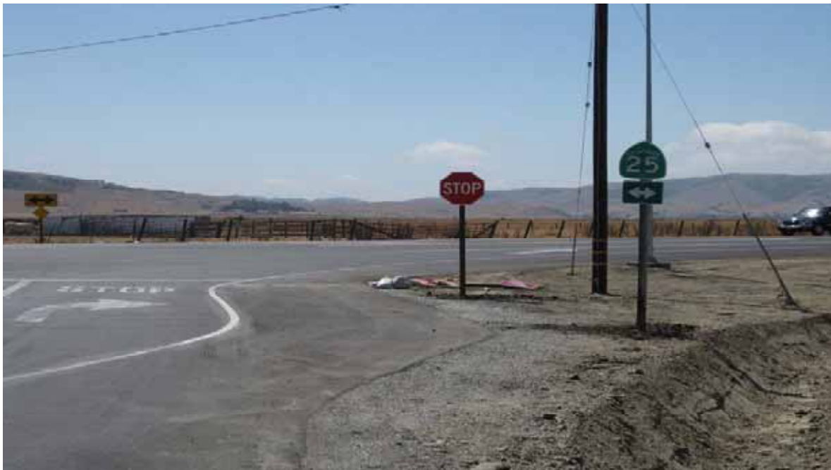
New Signs at Shore Rd Intersection
