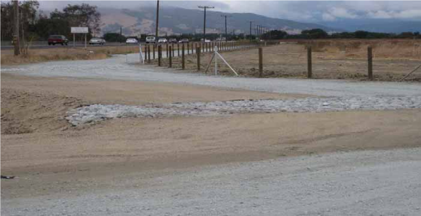
Stage 2 Fence @ Tri Cal
