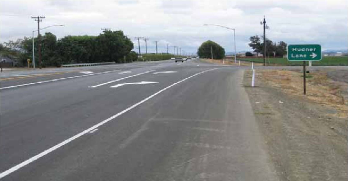
Intersection @ Hudner Ln. with New Signs
